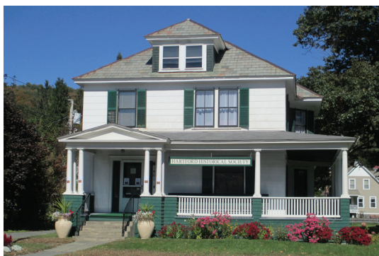
Garipay House with the restored roof front
