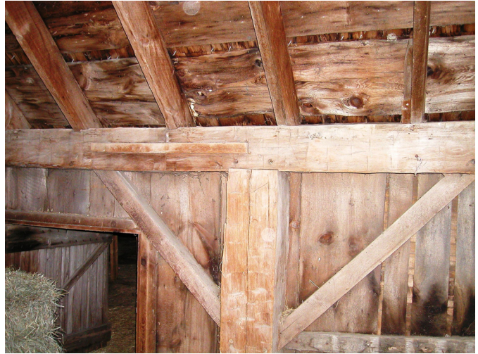
Milled rafters resting on hand-hewn timber in an 1840's enlargement of an earlier timber framed barn.
