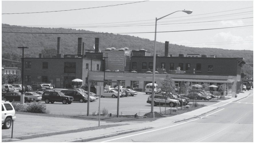
Tip Top “Complex” after renovations.
