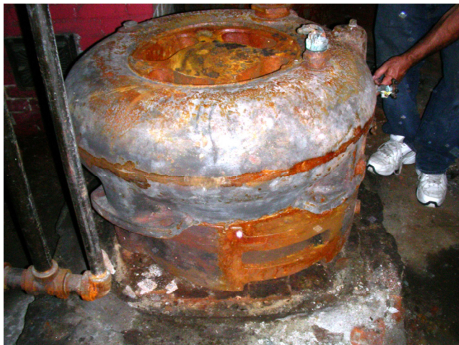
Boiler parts before demolition
