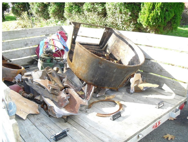
Boiler parts on truck before hauling away
