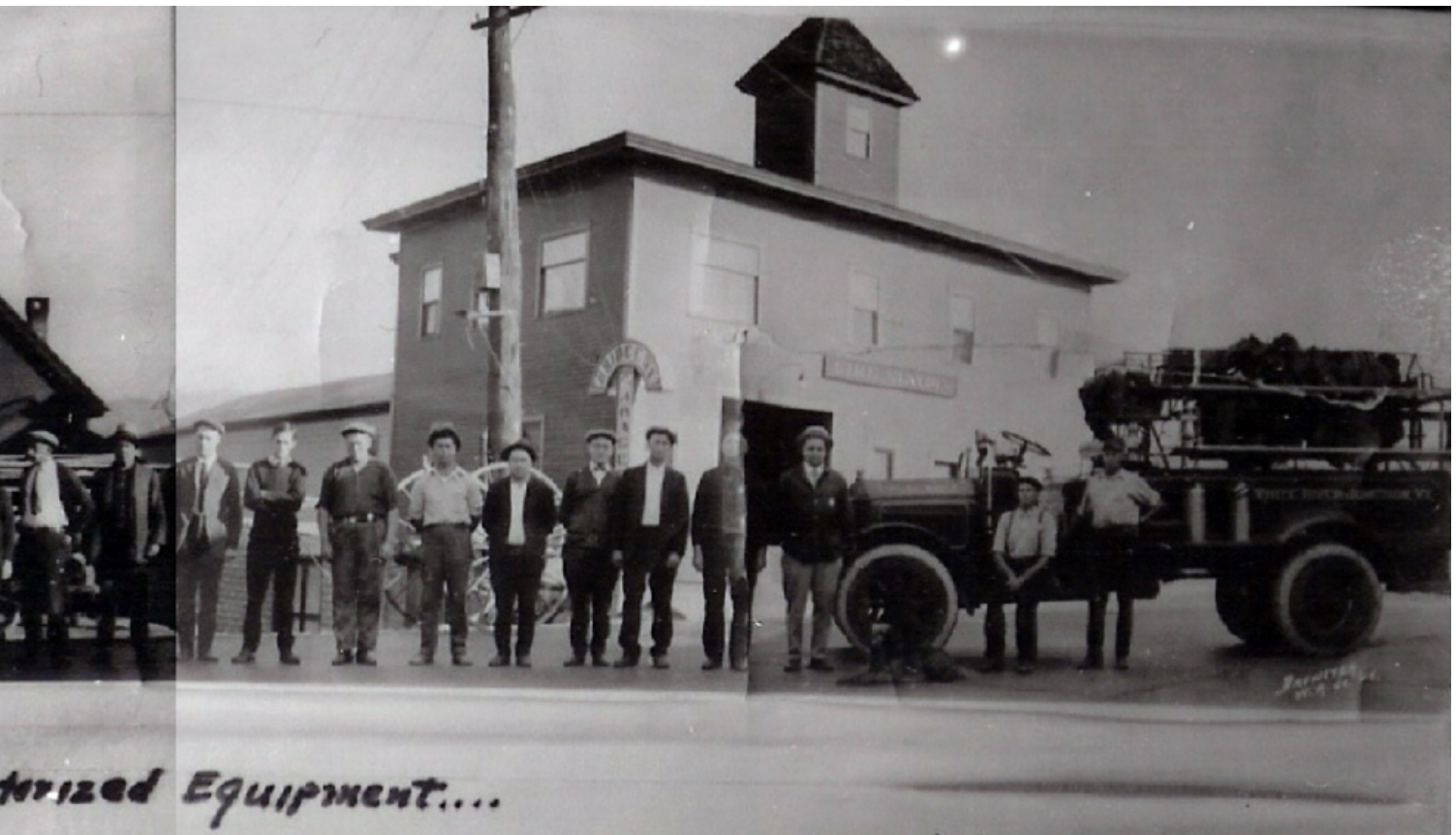
The Hartford Fire Department proudly displayed its Garford pumper truck in front of the recently enlarged firehouse in 1918. This was the town's first mechanized fire vehicle. A hose cart rests in the background.
