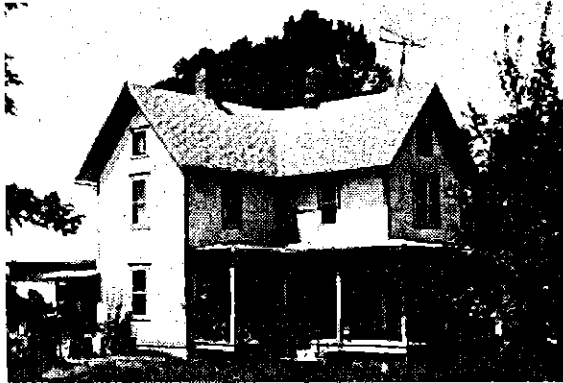
Typical Tri-Gable house of the period.
