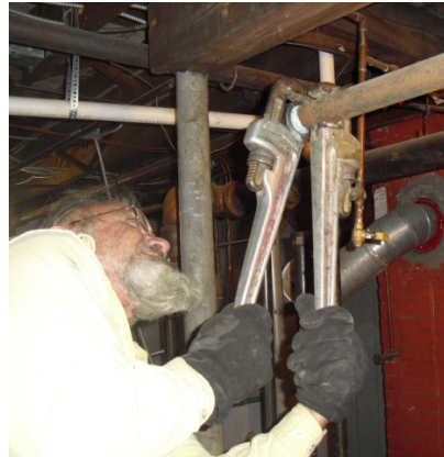
Brent Knapp installing new vents and fittings.
