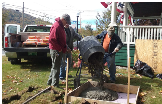
Brent and Gaylord mixing and pouring cement
