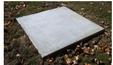
The finished base!
