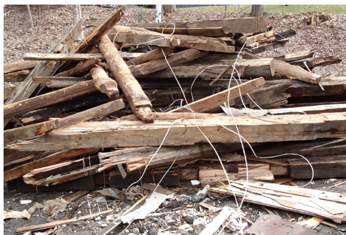
Top: Demolition was quick. Middle: The stone foundation exemplifies construction during that era. Bottom: Hand-hewn beams from the 18th Century.
