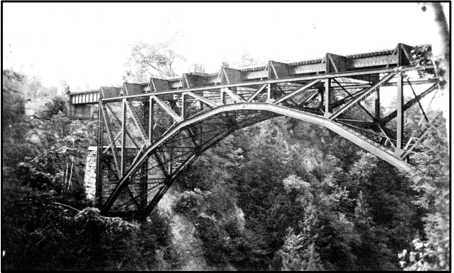
The completed Quechee Gorge Bridge Finished in the Fall of 1911 (Now US Route 4 highway bridge)
