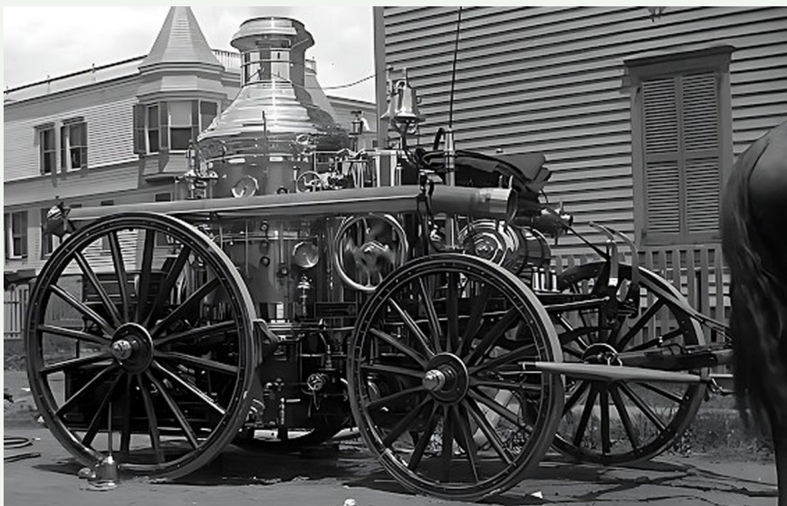
Hartford's first fire engine was a steam pumper built by the American Fire Engine Company of Seneca Falls, NY. The Vermont Standard reported that it was a Silsby-type machine, like the 1894 model above, that could pump 400 gallons of water per minute. The pumper was delivered to White River Junction in December 1893, and cost $3,000.
